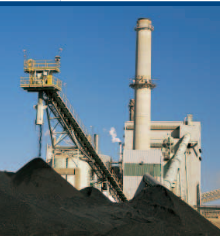
Counce's Multi-Fuel Boiler
